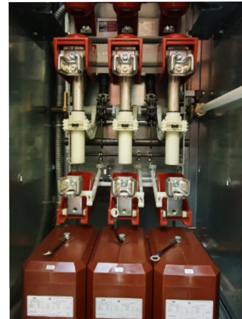
C3 shear load-break switches are usually integrated into the SAM. The switch-disconnectors formerly manufactured by ABB/Calor Emag are now produced by SZM.
