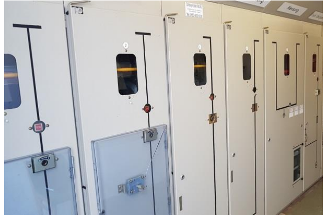
Switchgears up to 36 kV
